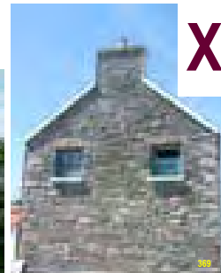
Poor practice - do not remove lime render to expose stone.
