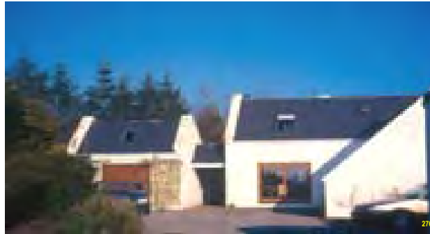
Raised concrete coping to gables
