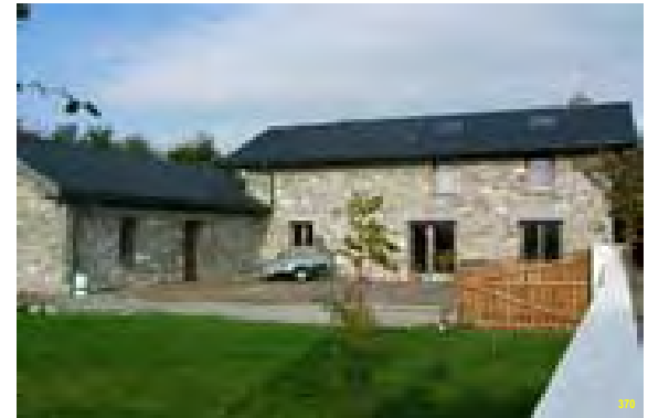
Poor practice - do not remove lime render to expose stone.
