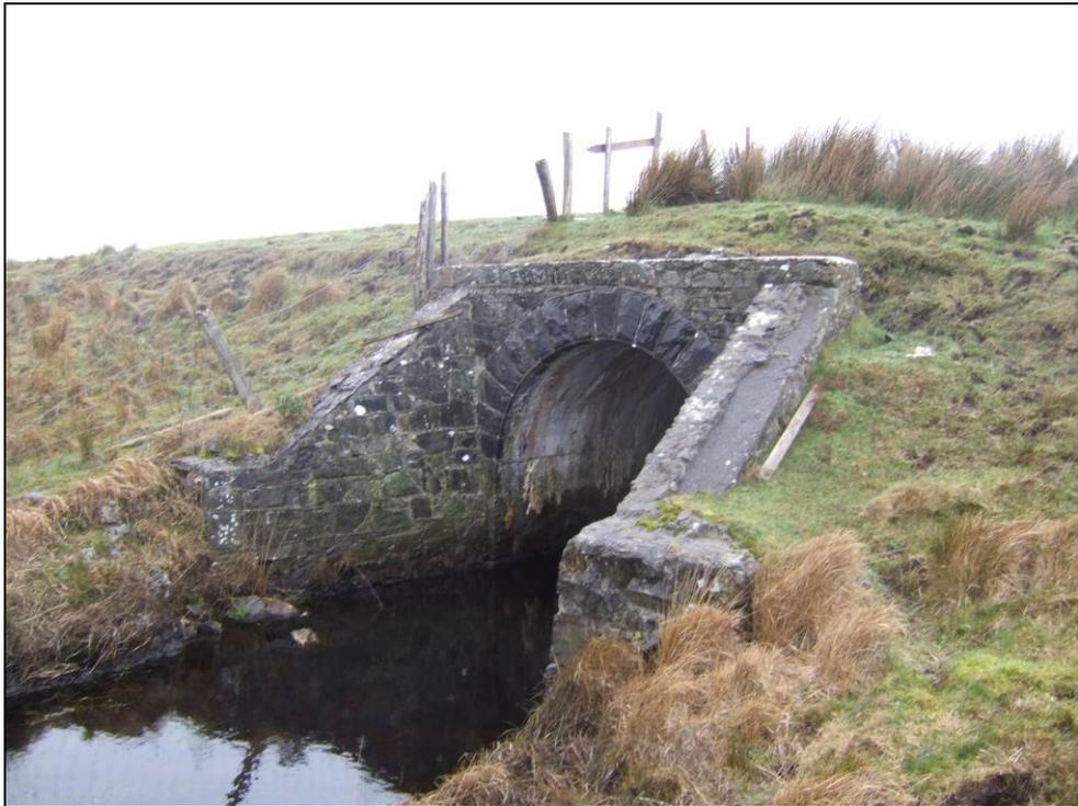
Plate 70 – BH 71, stone culvert/ accommodation bridge (Points 13-14), facing north-west
